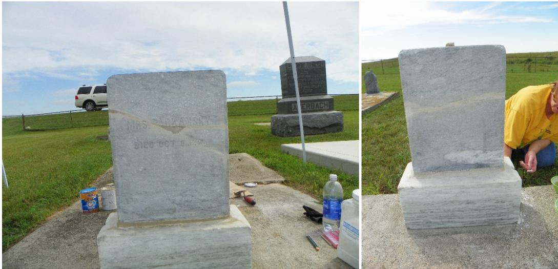
**Figure 7. The Parkansky marker after Lithomex application (front and rear. The center was still damp and had not dried yet. Humidity on site averaged 80% affecting dry time for both Lithomex and Rivo 50.**
